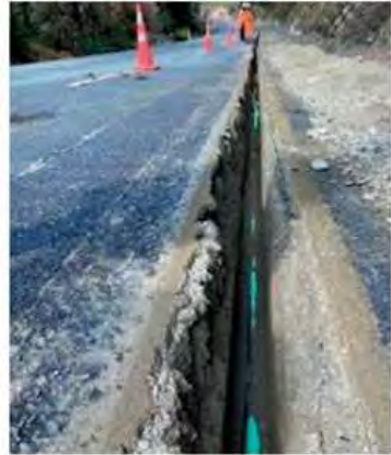
Trench ready for backfill and re-instatement of the road surface.
