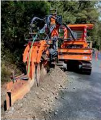
Rock saws cutting a road trench and installing the Chorus green duct ready for fibre.
